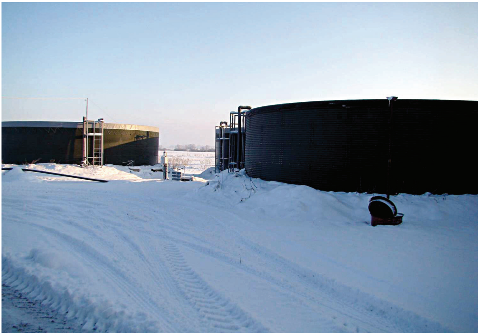
FIGURE 11.2. Cement slurry container
